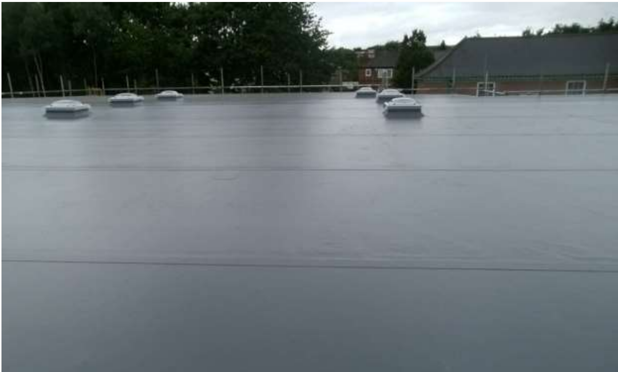
Example Roofing: EPDM roof
